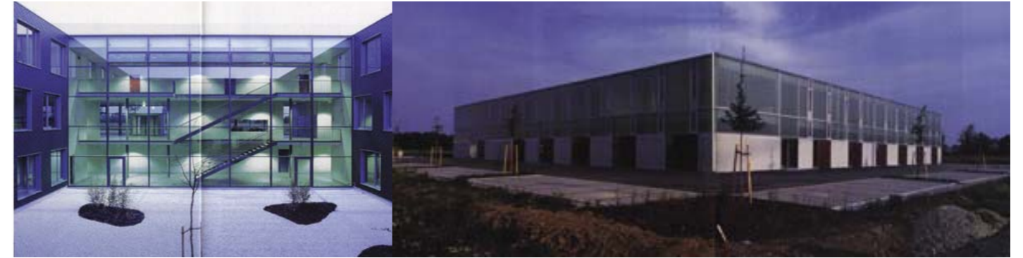
Development Centre, Ingolstadt, Fink & Jocher, Munich
