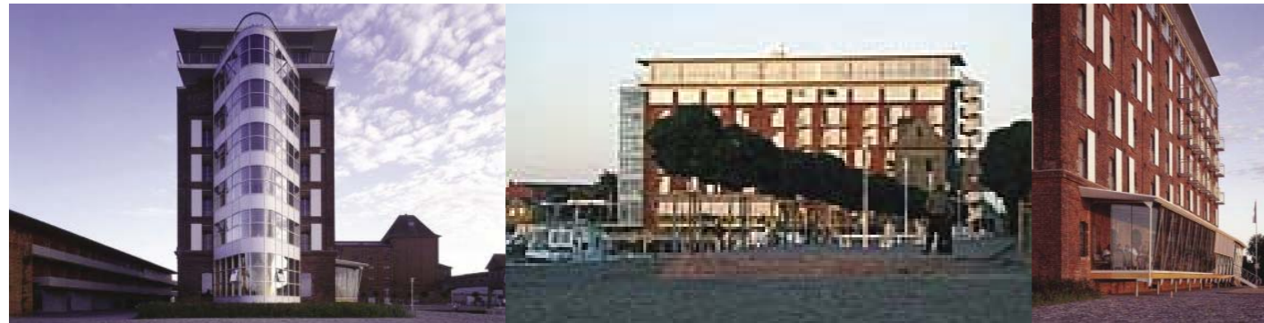
Granary Hotel, Barth, Germany, Giencke & Company, Graz, Austria
