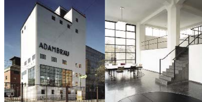
Architecture Centre, Vienna, Conversion of an old brewery, Giner & Wucherer with Rainer Körberl, Innsbruck, Austria
