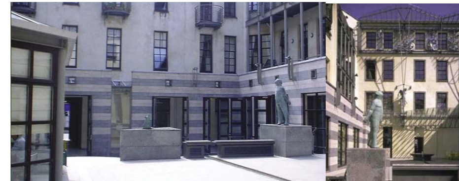
Italian Centre, Glasgow, Page & Park, Glasgow, UK
